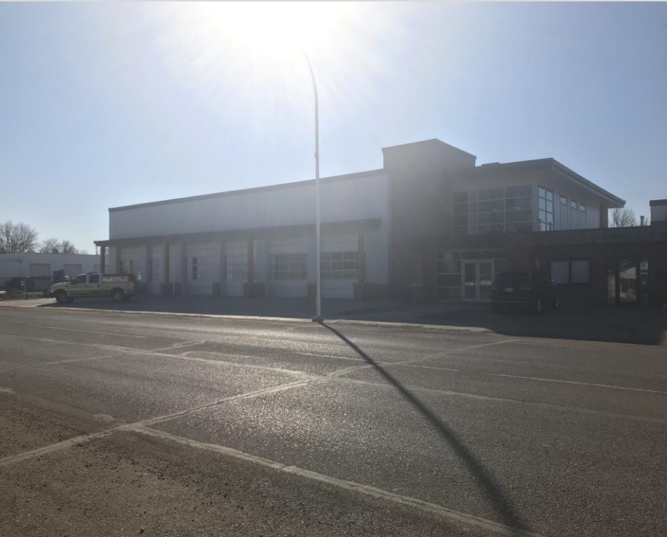
Phase One firehall construction
